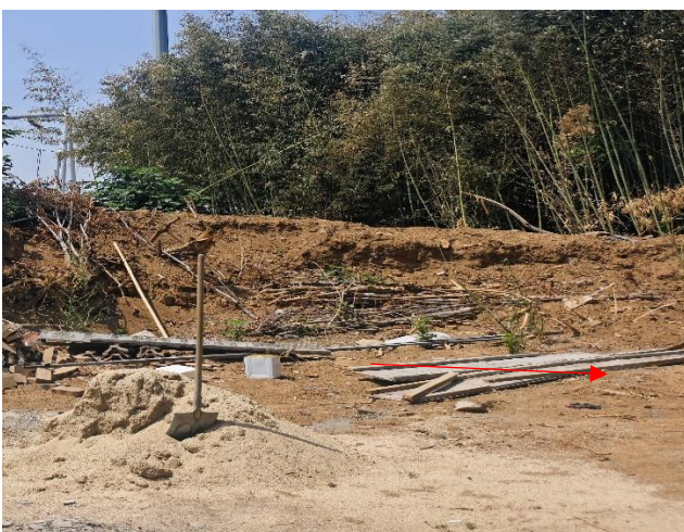
110kV薛村站东侧50m处~110kV薛村站单回电缆北侧衰减
